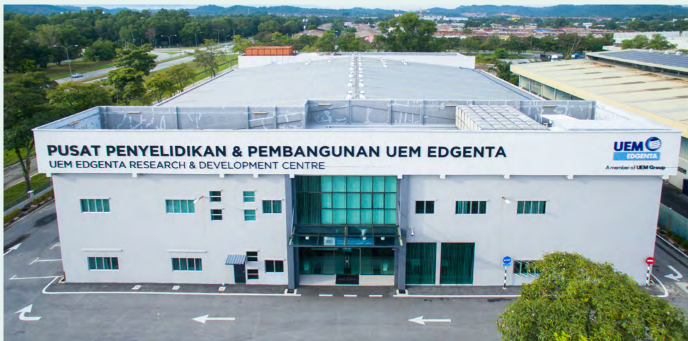
UEM Edgenta's Innovation Hub, The Pavement and Research Centre
